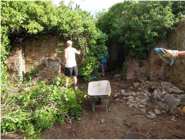
Figure 10: view from inside TDV 1 in the direction of the entrance of TDV 2 in 2014.
