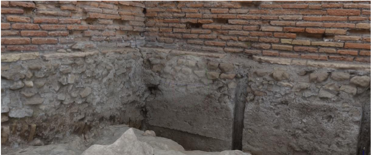
Fig. 3 The fundaments of the northern wall (on the right) and the western wall (on the left)
