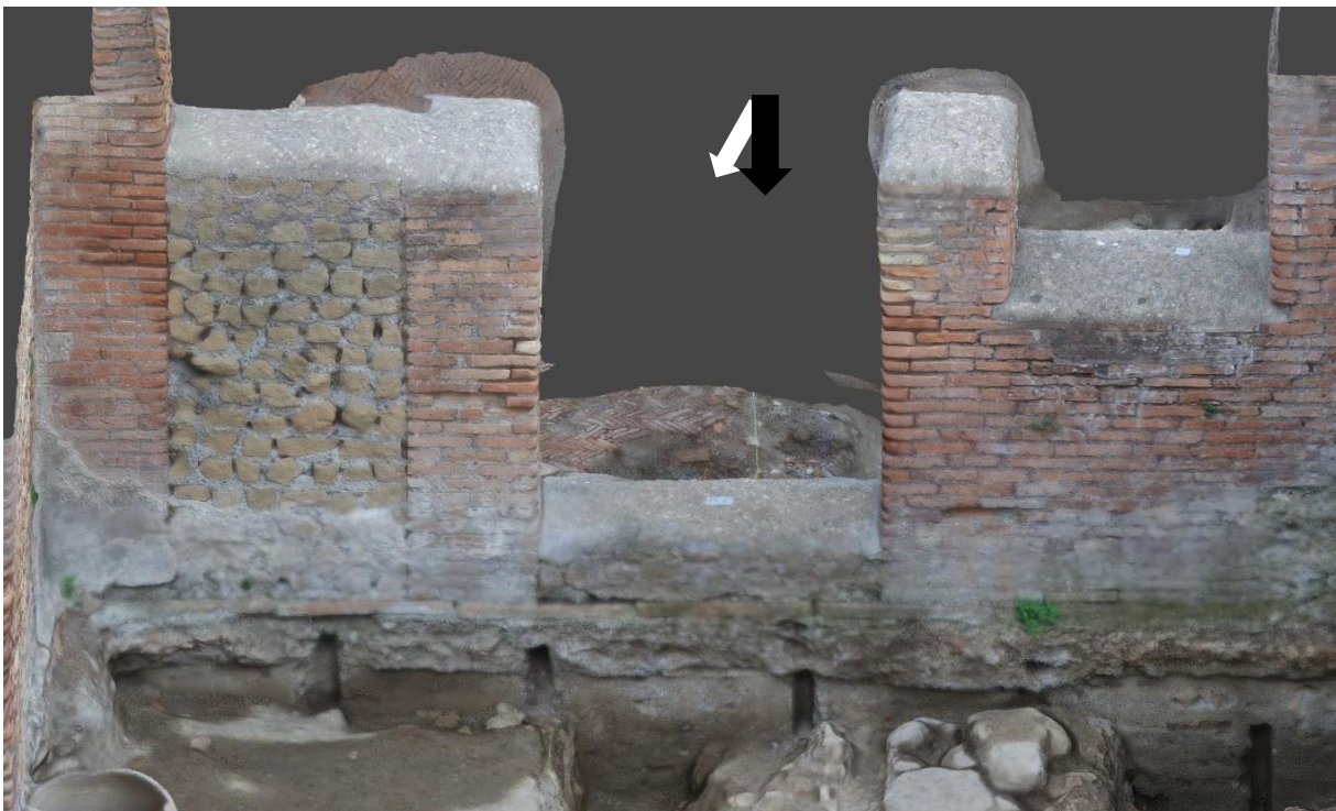
Fig. 4 The southern wall of the area TFR2 with the once closed-off wall towards the area TFR1
